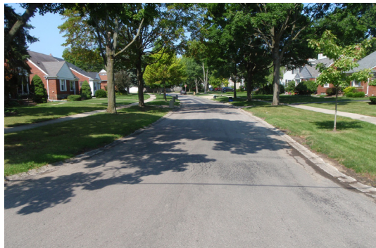
Unimproved Road with Gutter
